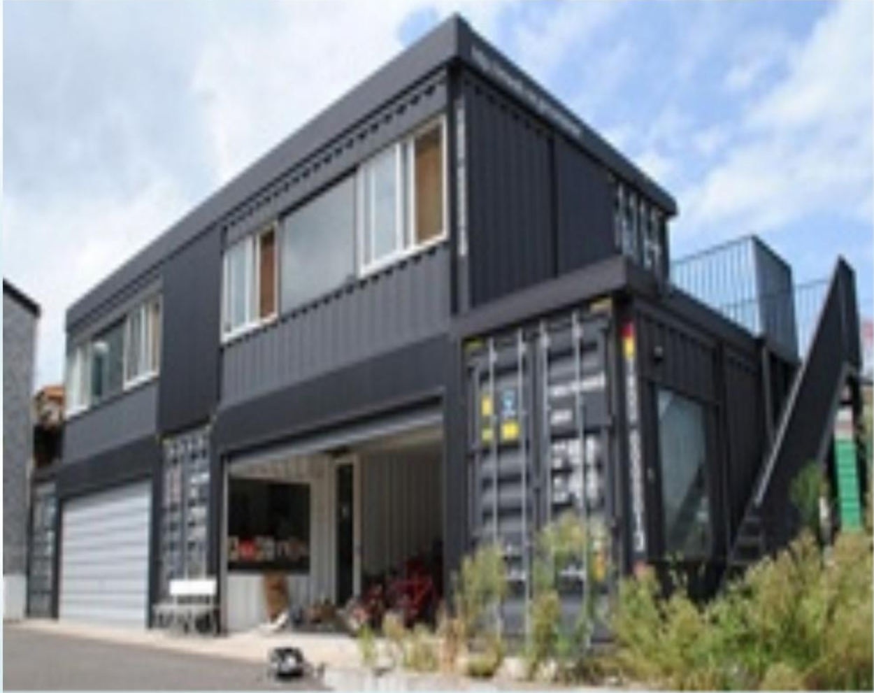
Photograph 3 A transport container converted into storey house .Source, adopted by researcher from Google scholar (2019)
