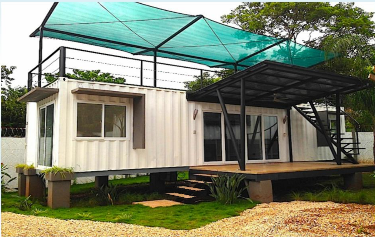
Photograph 2. Transport containers converted into self-contained house. Source, adopted by researcher from Google scholar (2019)
